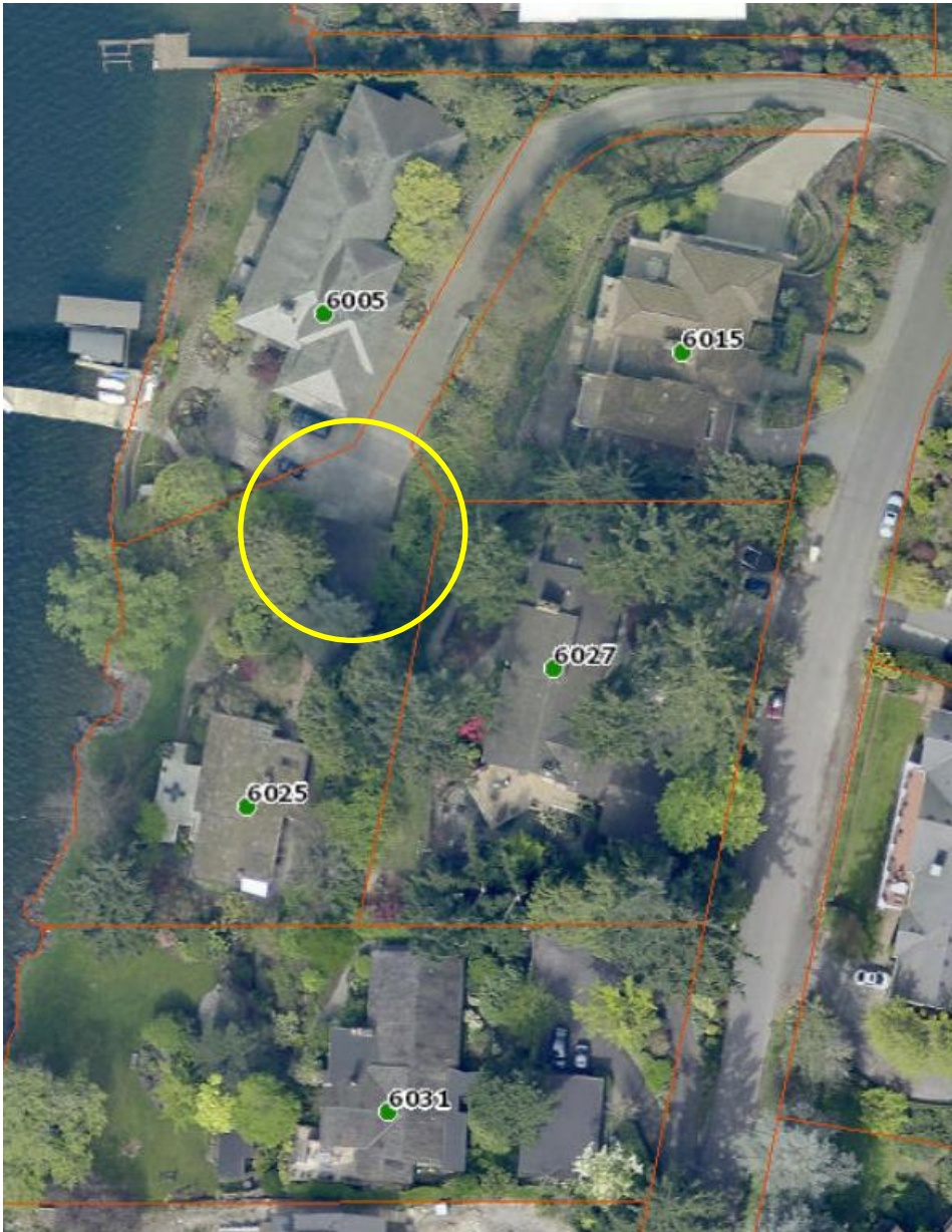
Figure 1. Aerial overview of the subject (6025) and surrounding properties. Note the carport sits directly in the center of the only viable approach to the property (yellow circled area). The entrance is only 75' wide at this point, 15' of which is close vertical along the east side.
